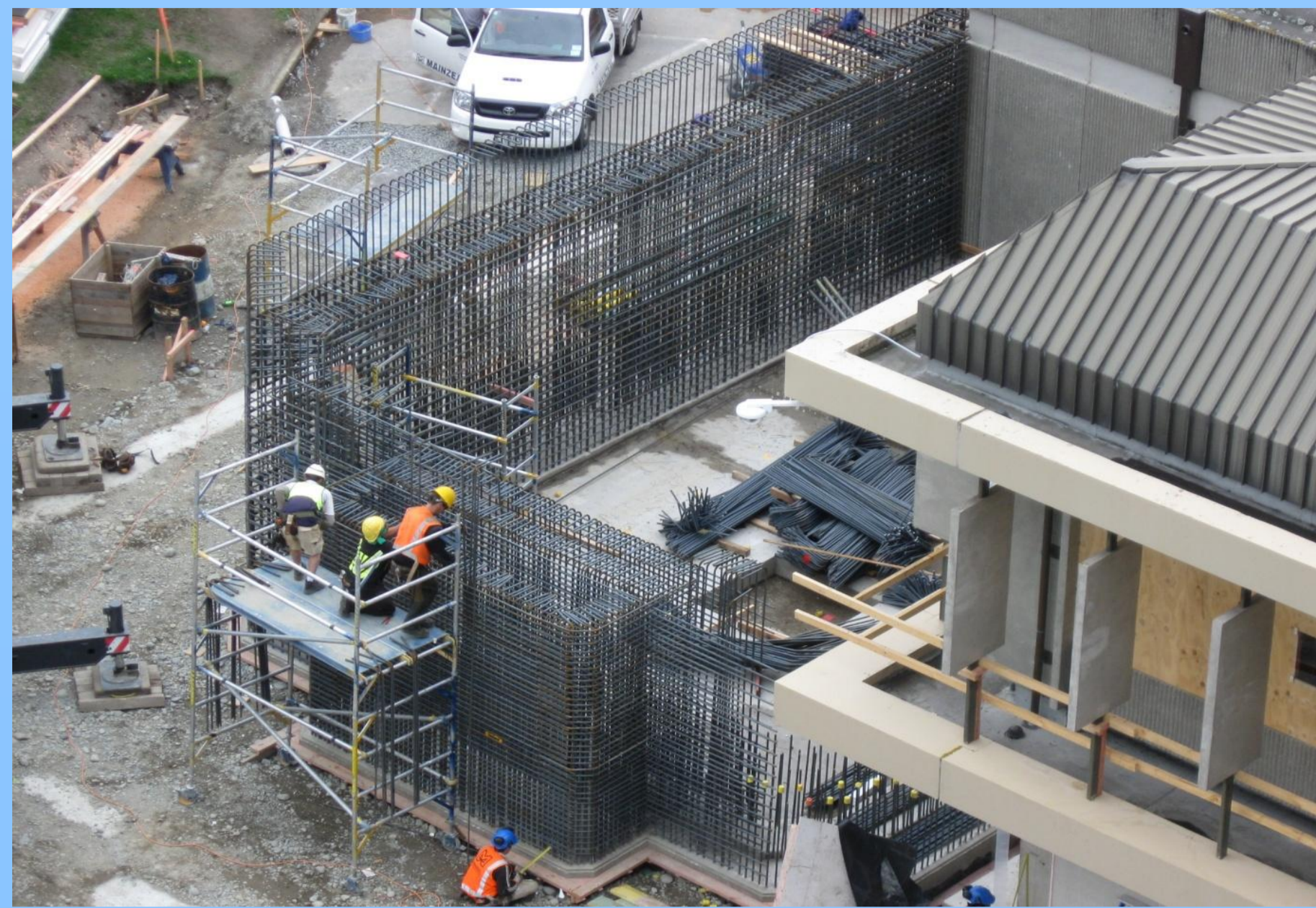
Photo 1 - Steel reinforcing also present in concrete walls
