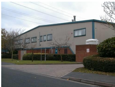
Figure 5: Radio-chemical facility building prior to remediation
