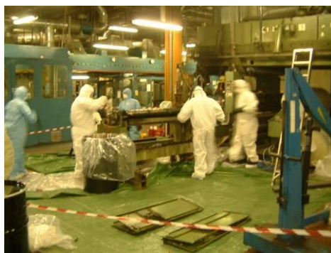
Figures 3 and 4: Decontamination of industrial plant
