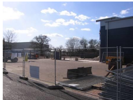
Figure 18: Final site clearance
