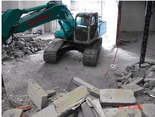
Figure 9: Remediation of building
