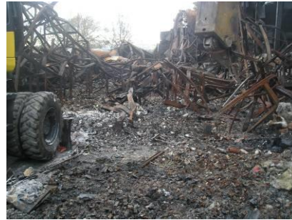
Figure 12: Remains of warehouse and contents
