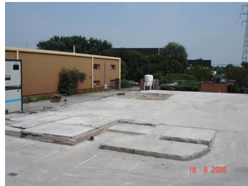
Figure 10: Base slab of building post remediation
