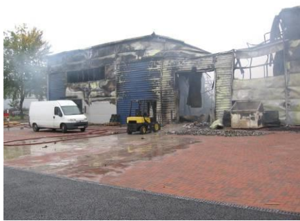
Figure 15: Warehouse after fire extinguished
