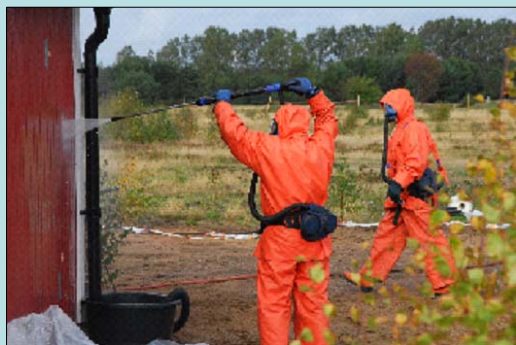
High pressure hosing of a radioactively contaminated wall in connection with a Nordic preparedness exercise in 2007.
