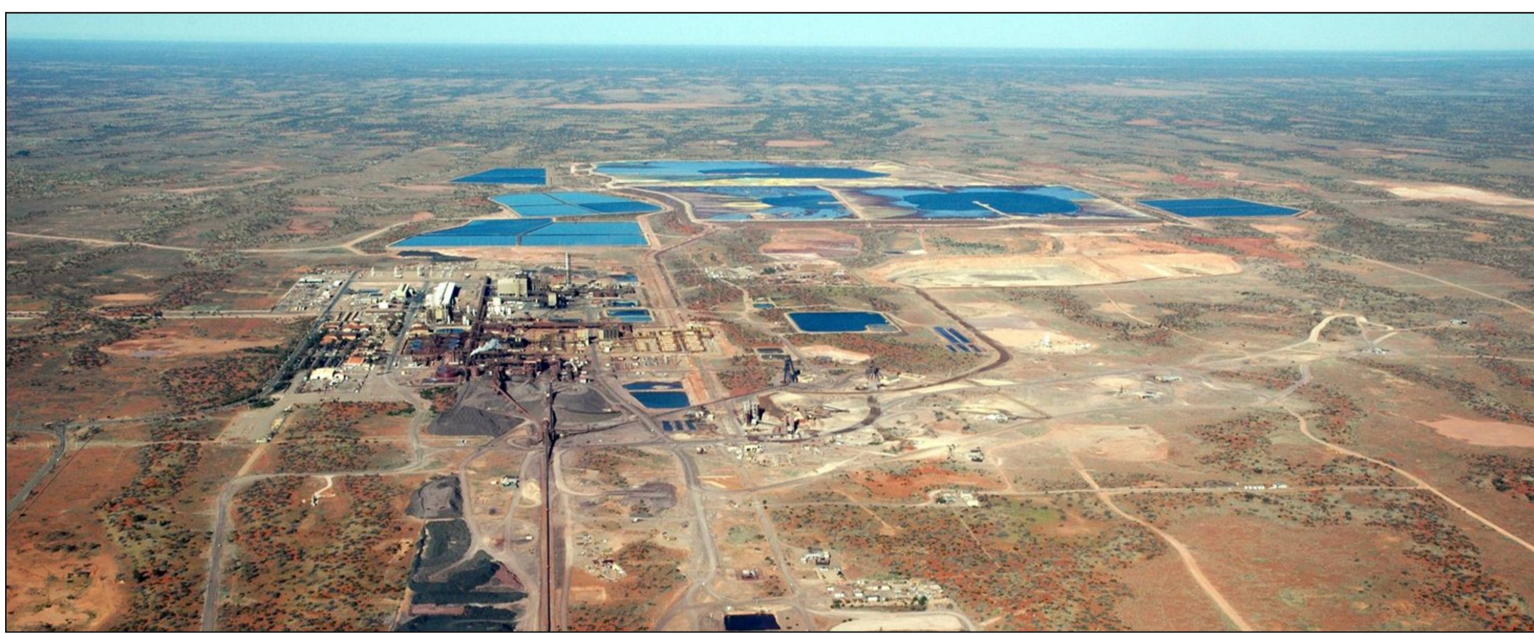
Figure 2: Aerial view of current Operation
