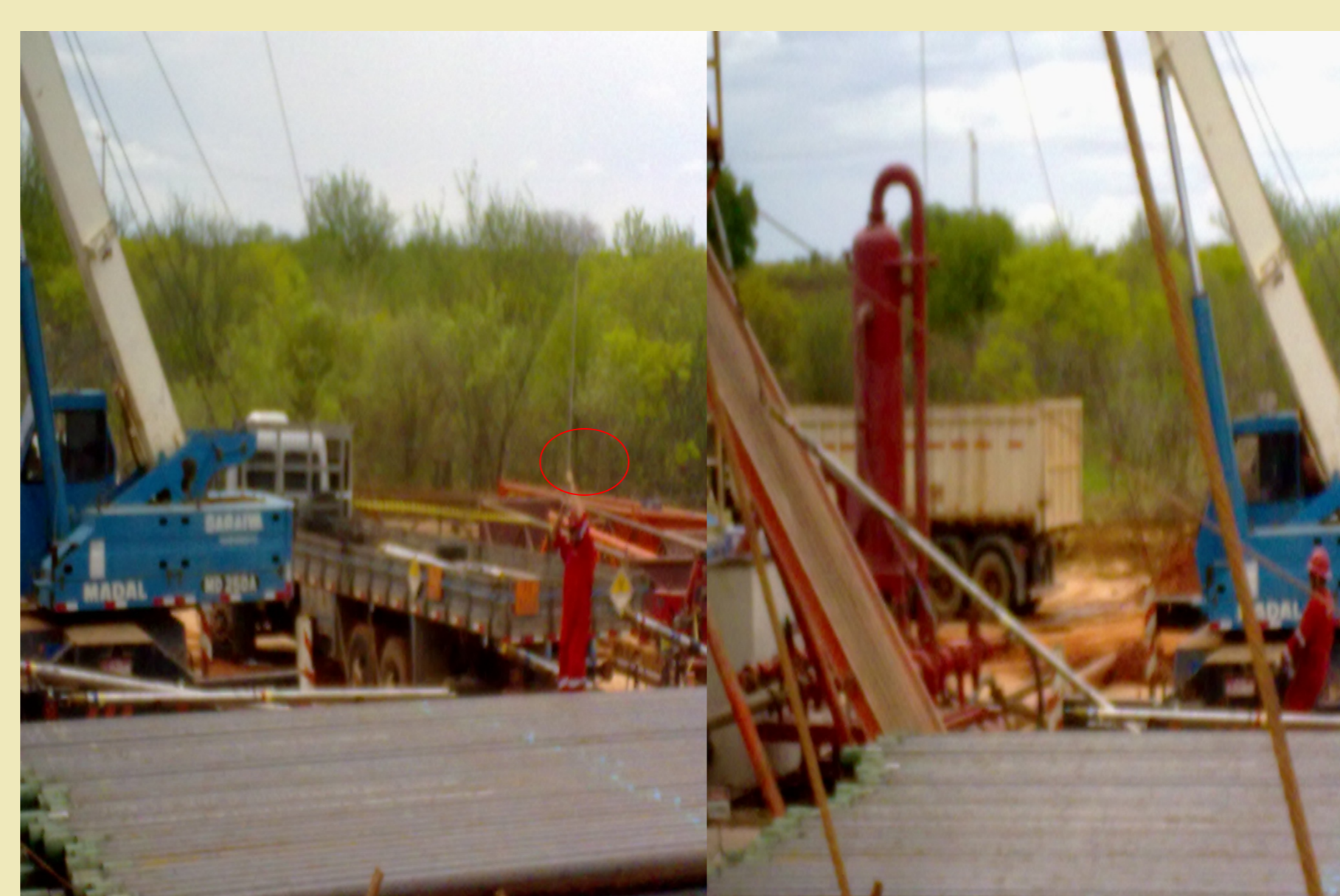
Figure 3 – Procedure 2. The radioactive source (red circle), was removed of this shielding below the rig floor level.
