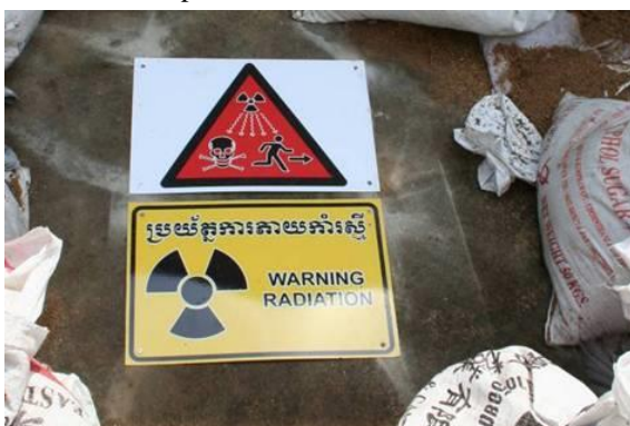
Figure 10: Warning sign installation on top of existing concrete slab and sand infill.
