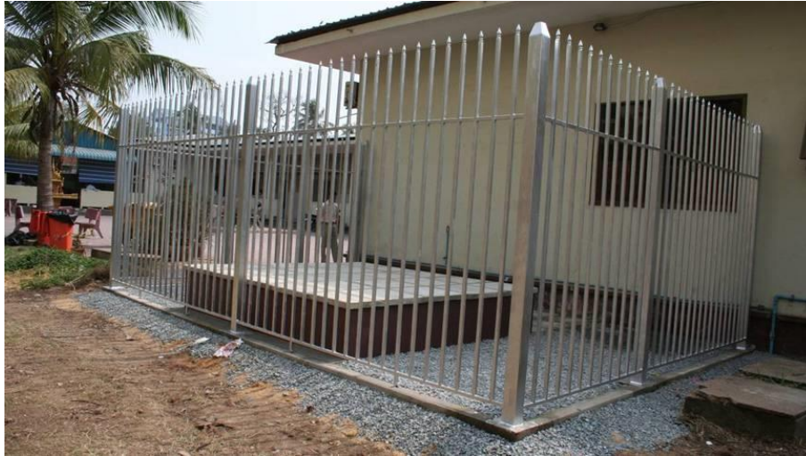
Figure 11: Site after completion of improvement works.
