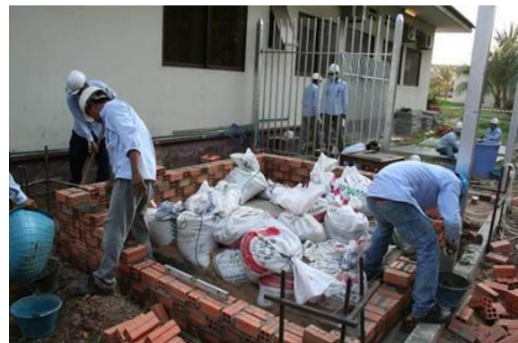
Figure 9: Brick work for the shielding enclosure and concrete infill up to the bottom concrete block.
