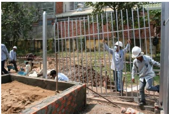
Figure 8: Installing the security fence and gate around the hospital buried source site.
