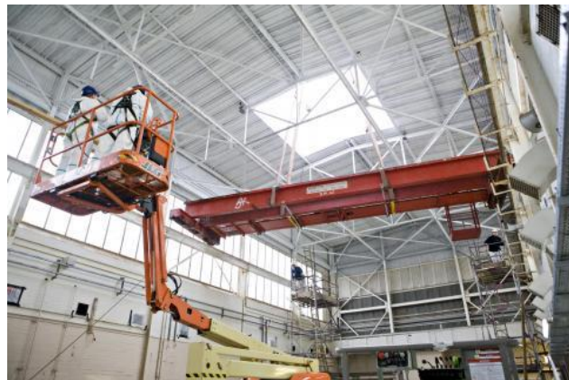
Figure 8(b) Decommissioning team removing services
