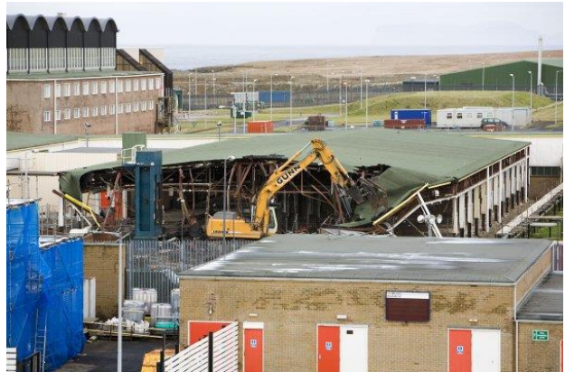
Figure 7(b) Demolition of fuel fabrication plant
