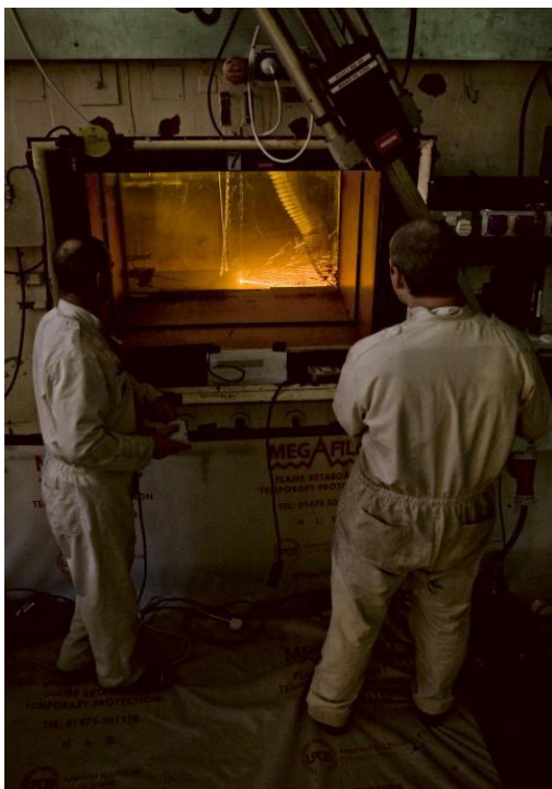
Figure 10(a) Plasma cutting in D1217
