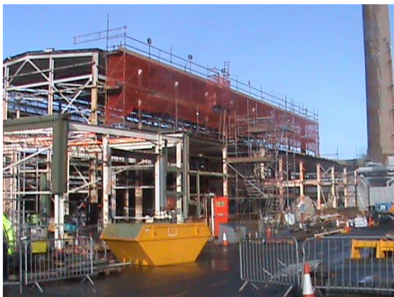
Figure 8(a) D1207 Prior to demolition
