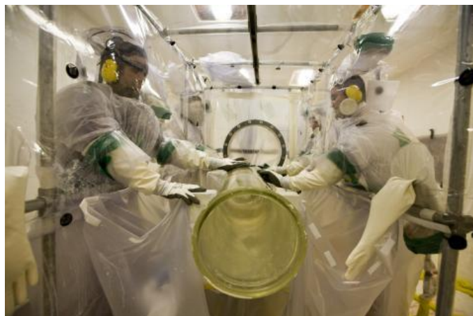
Figures 15(a) and 15(b) A two-piece Air Fed Suit being worn during decommissioning activities
