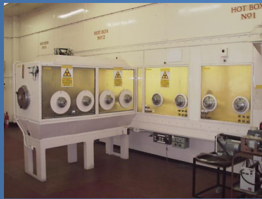
Fig 1 – Typical Boxes at Project Start
