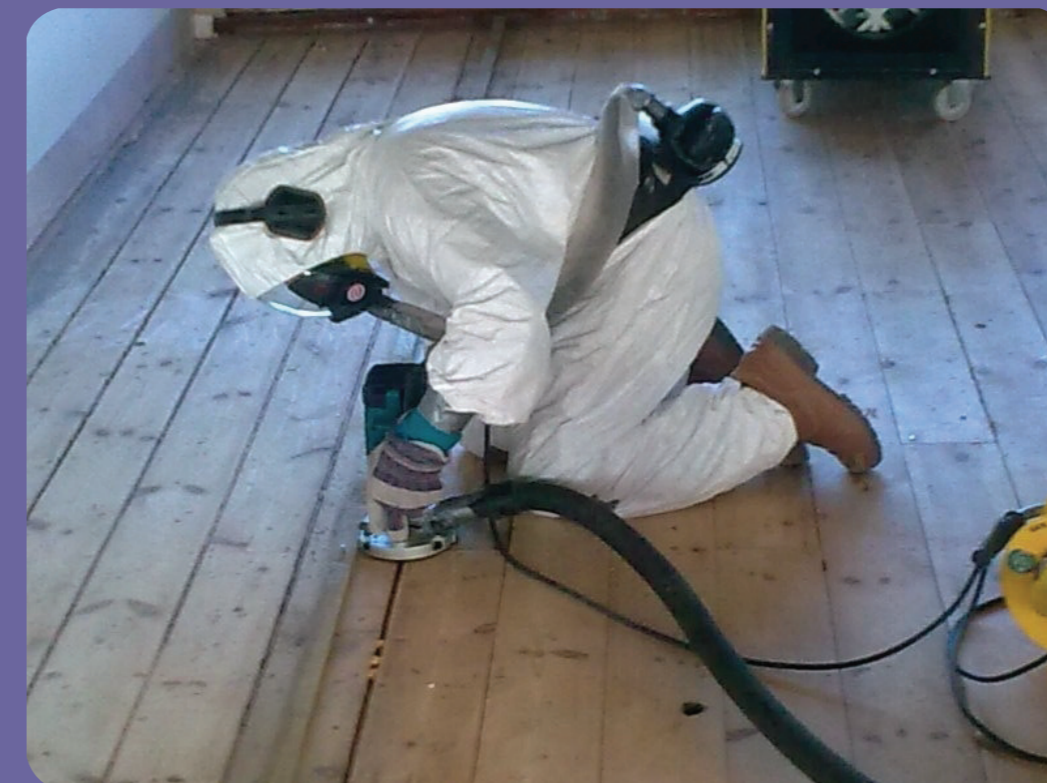
Fig 2: Remediation of wooden flooring
