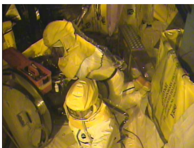
Figure 4 - SG primary side platform work area
