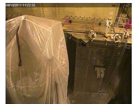
Figure 7 - Upper Cavity Decontamination using RM1 Wall Cleaner suspended from the Polar Crane
