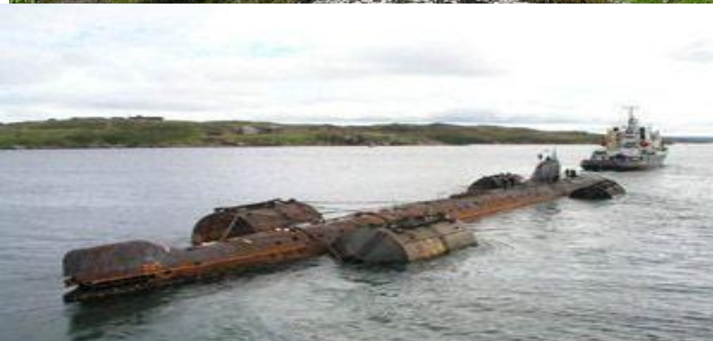
Nuclear submarine dismantling
