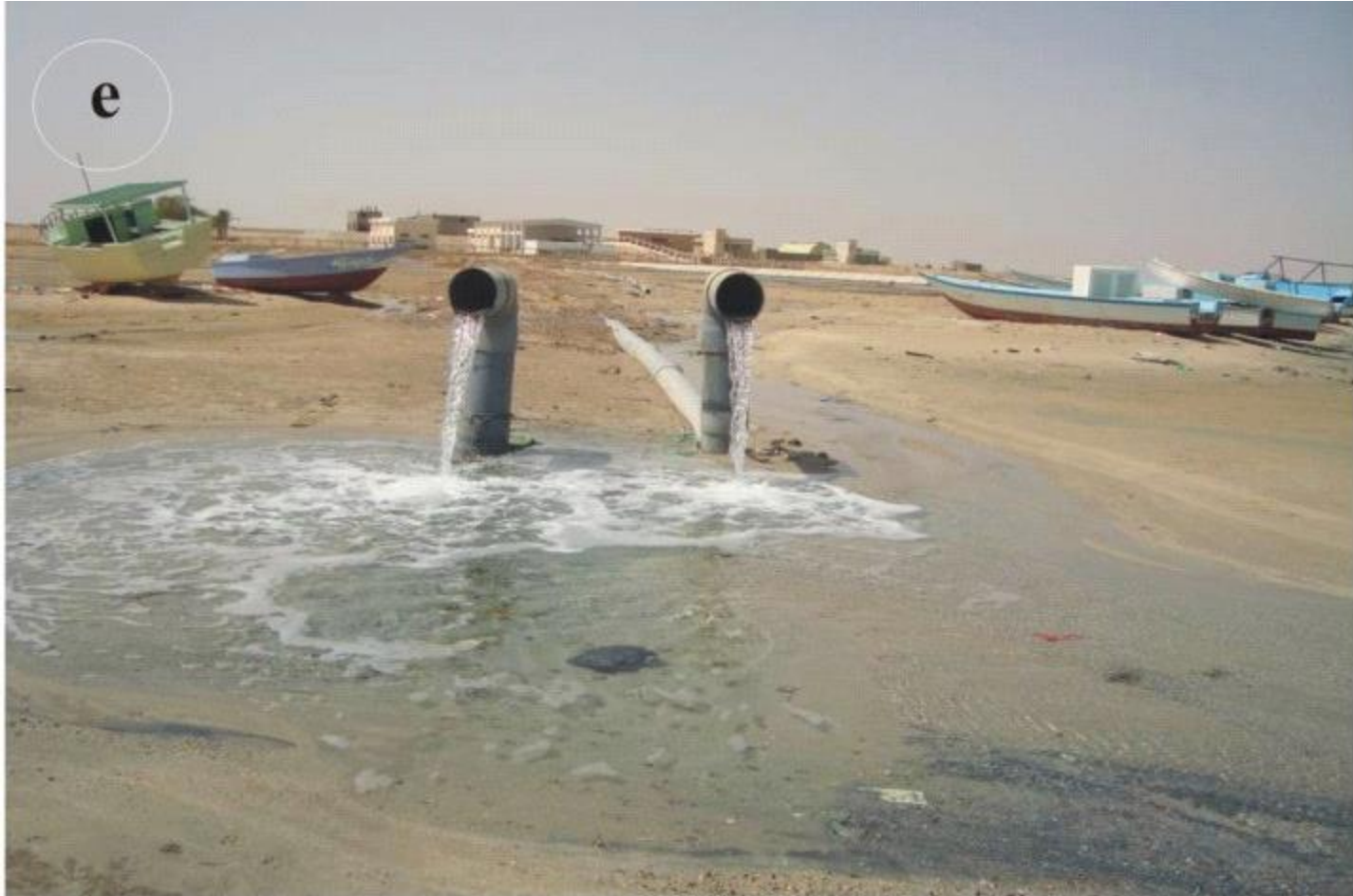
drainage of reject water of desalination water plant
