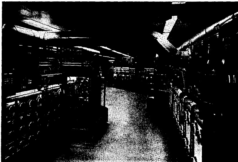
FIG. 1. A view of the ANL fuel fabrication facility glovebox system.
